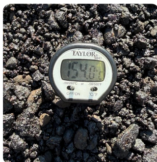
Mix temperature at laydown
