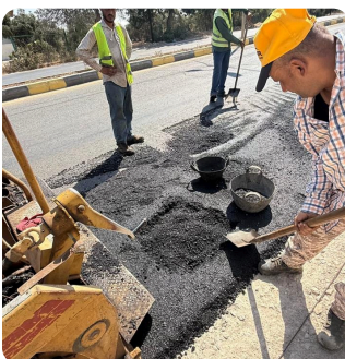
Sampling the asphalt mix behind the paver
